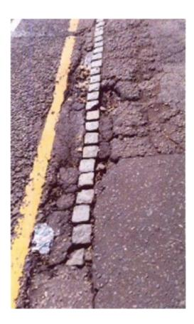
The highway authority immediately carried out temporary repairs, with more permanent repairs following in 2017 and 2018. The parties' experts agreed that the pothole was about 200mm wide, 200-300mm long and 40-50mm deep.
